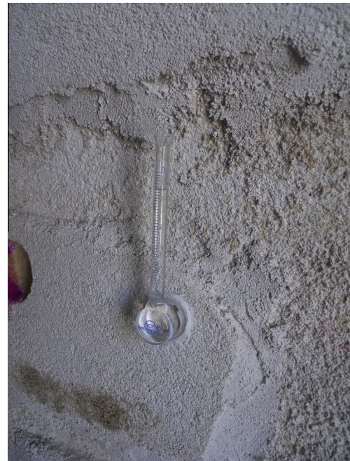
Fig. 15. Demonstration of Karsten tube testing on mortar.
